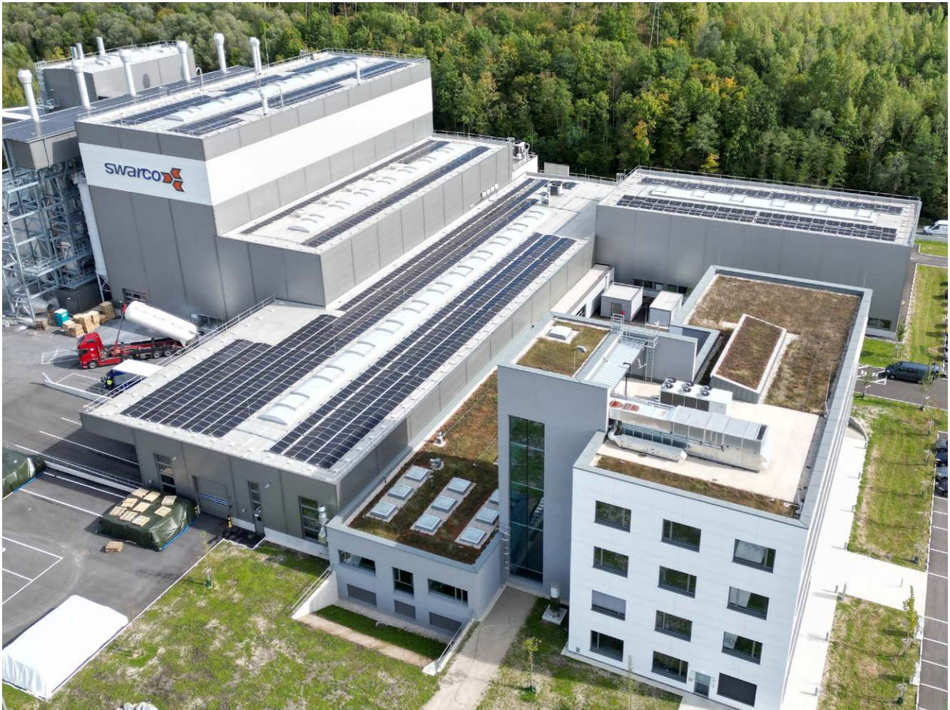
Photovoltaic system at SWARCO Global Glass Beads Technology Center
